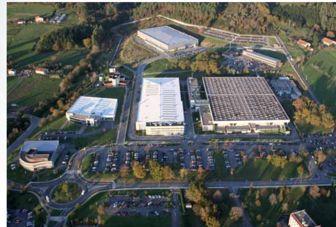
The main headquarters of ITP in Spain
